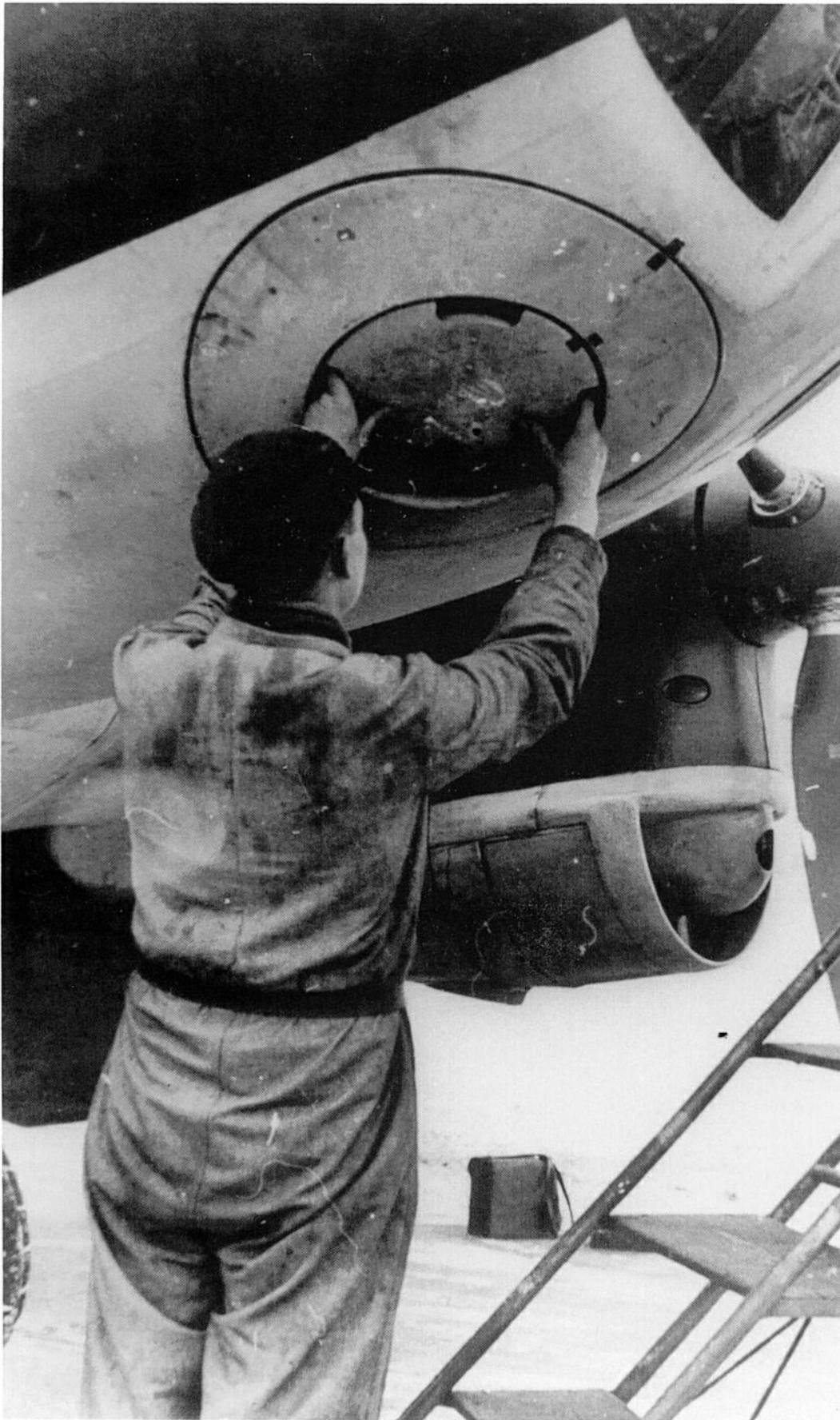
Left: This Ju 86 P-1, probably the V 2, was tested by the VfH (High-Altitude Research Establishment) at Oranienburg. The screwed access hatch for the two-seat pressurised cockpit is seen here.
