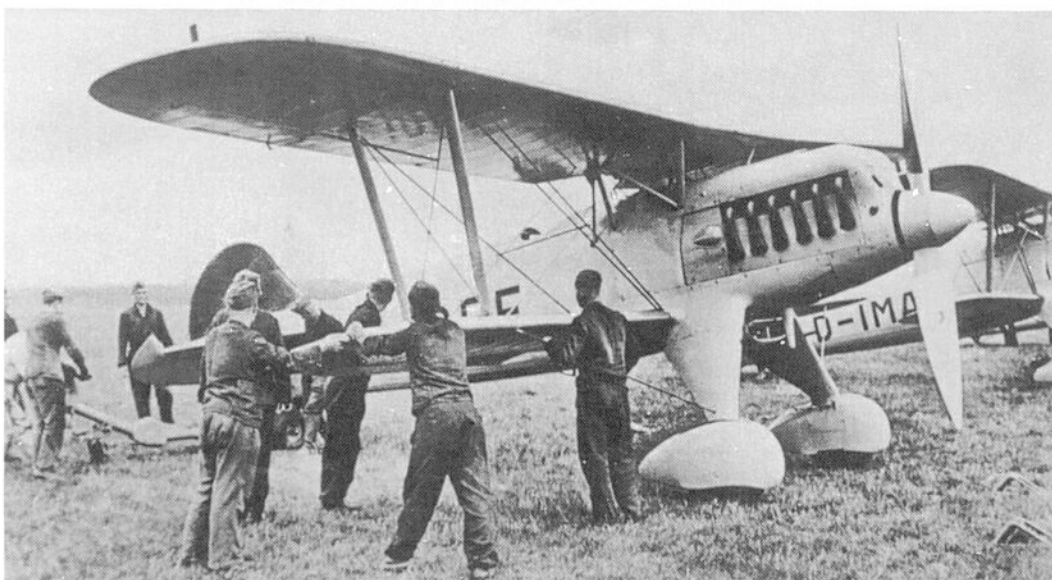
Left: The Heinkel He 51 was, with the Ar 68, the first standard fighter of the Luftwaffe. The first zero-series aircraft carried the registration D-IQEE.
