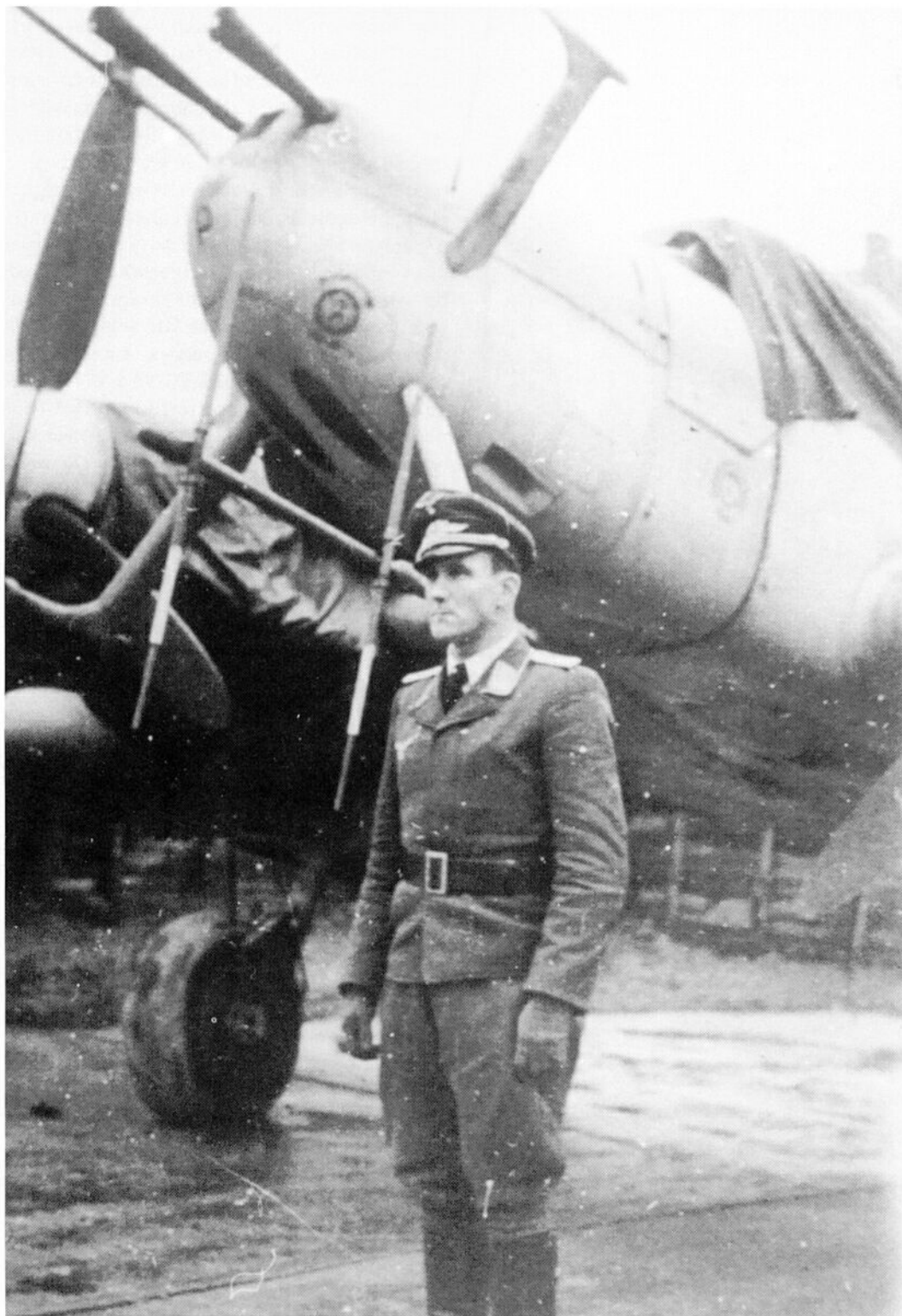
Left: The Bf 110 G-4/R4 had four nose-mounted MG 151/20 cannon in place of two MK 108s. This aircraft, seen in the summer of 1944, was attached to 5./NJG 5.
