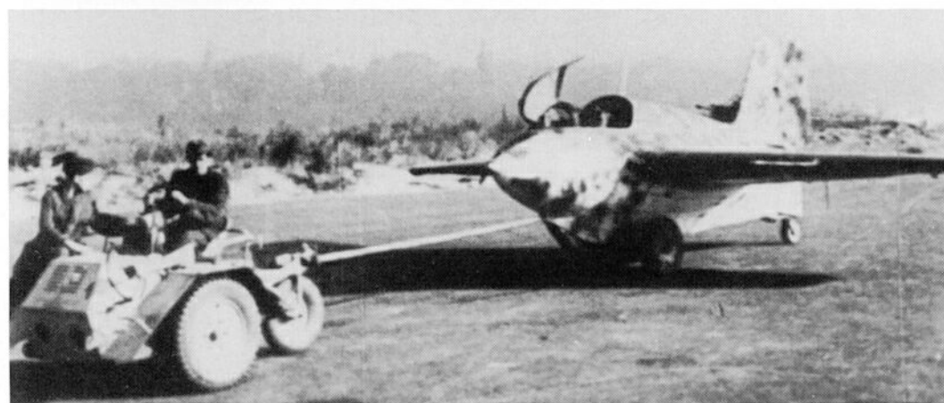
Left: For the Me 163 a special vehicle, the 'Scheuch-Schlepper', was developed.
