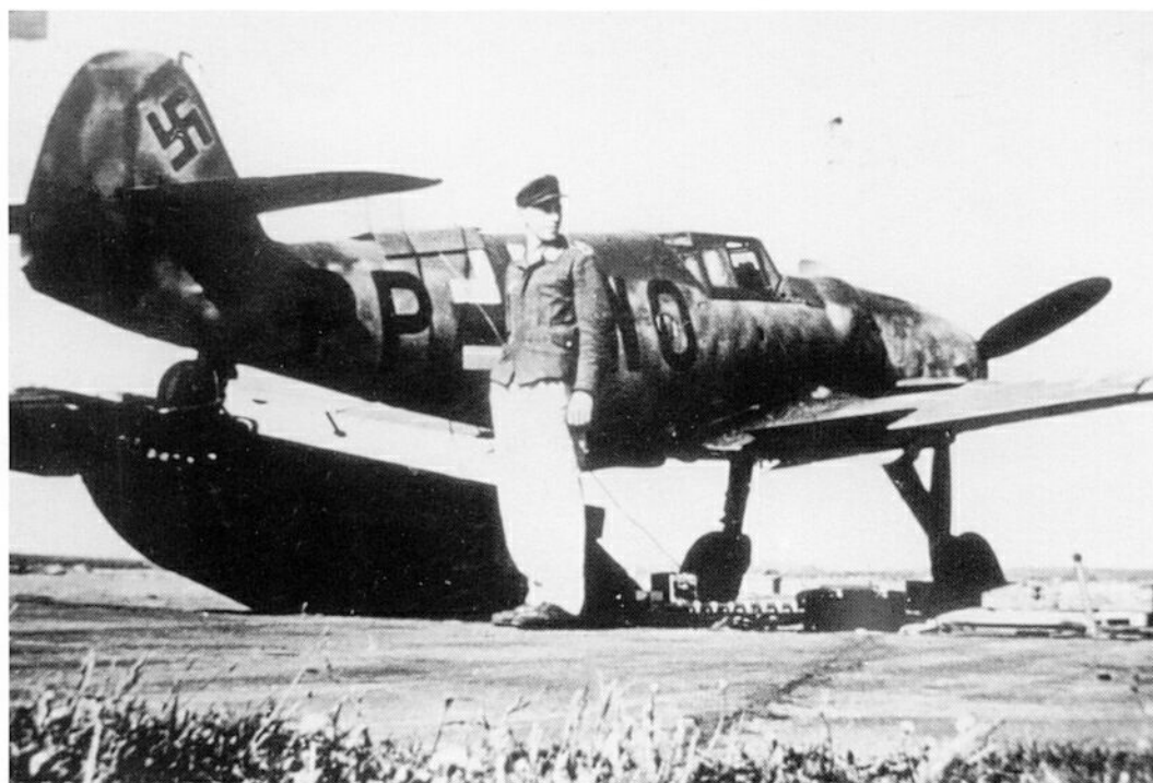
Left: A small number of Bf 109 G-6s were equipped with the FuG 217 'Neptun' radar as part of the 'Wilde Sau' (Wild Boar) night fighter campaign.
